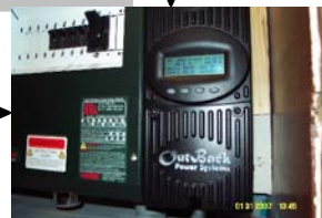
Wind Turbines Feed Battery Charge Controller.
